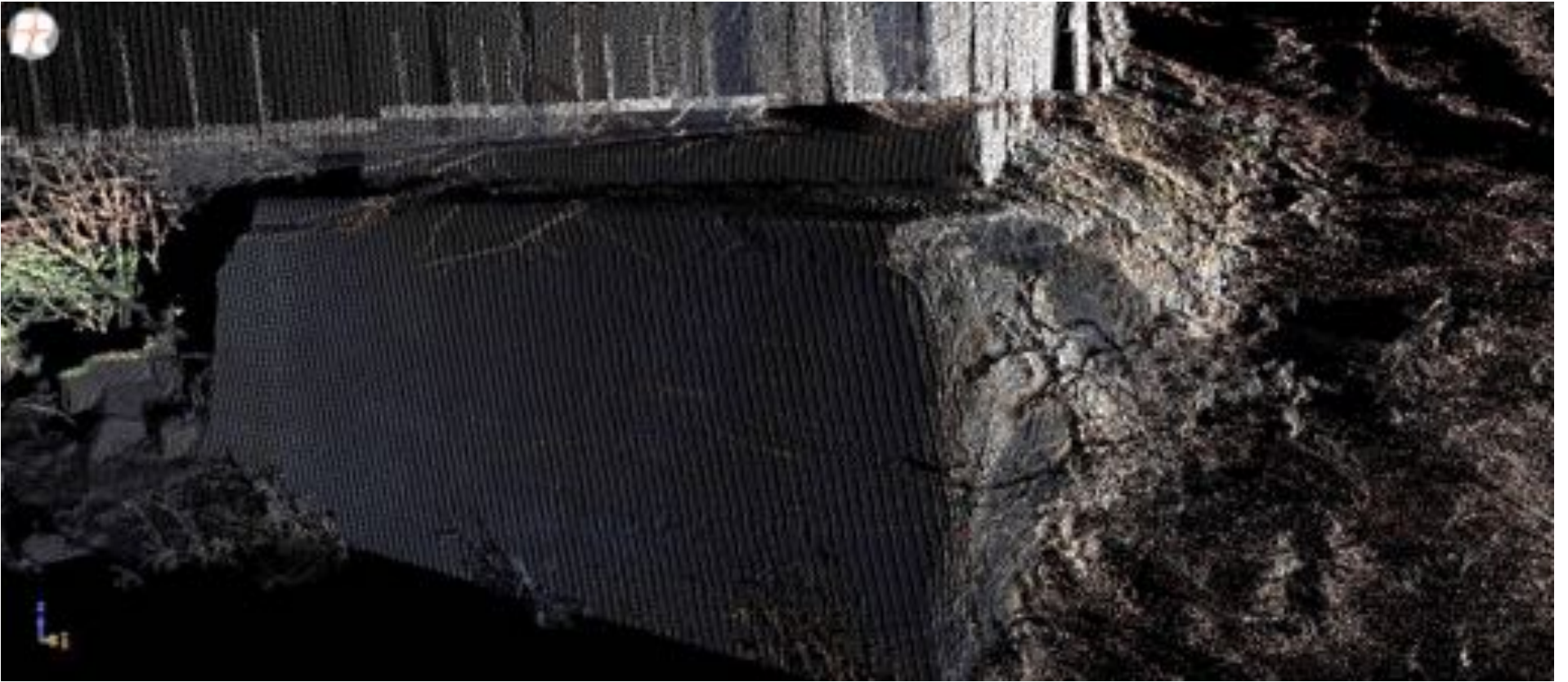
Quinlan Covered Bridge Abutment, Charlotte, VT
